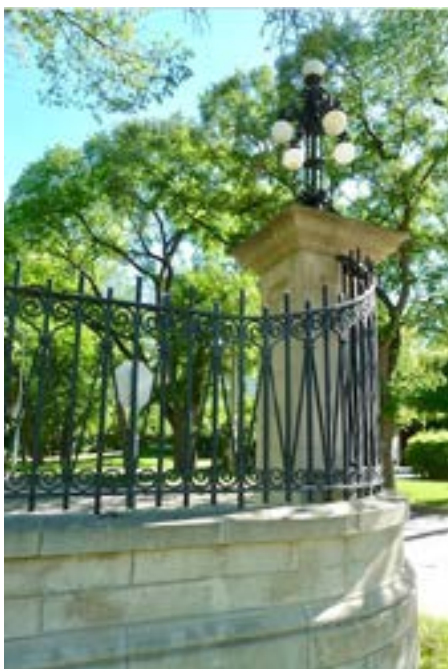
The larger pillars are set farther back than the smaller ones, creating a graceful curve in the limestone base and wrought iron.
