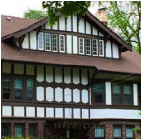
131 West Gate, 1912 - the hallmark of Tudor style is its half-timber detailing (strictly ornamental these days) with stucco or stone infill.
