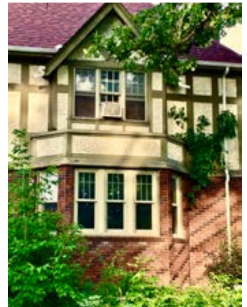
12 Middle Gate, 1929 - classic Tudor windows are narrow, tall, multi-paned and are clustered together. Note the love of detail in the window surround and the house’s patterned bricks.
