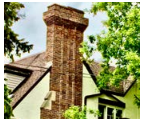
6 Middle Gate, 1912 - a massive Tudor chimney with more decorative brickwork.
