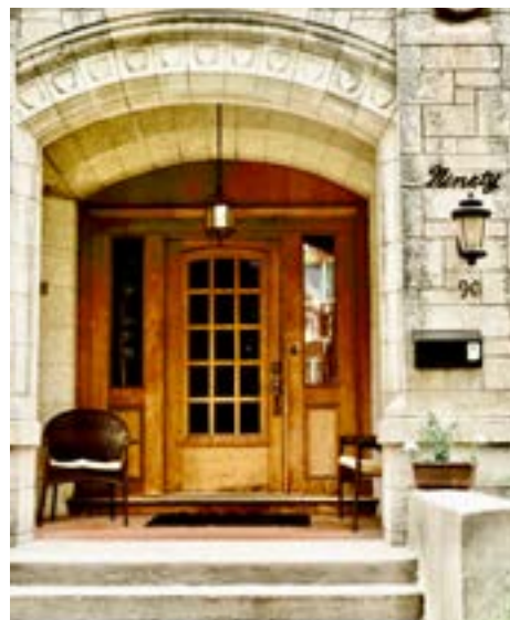
90 East Gate, 1909 - arched doorways are a common feature of Tudor-style homes, often with ornamental surrounds that lend prominence to the entry.
