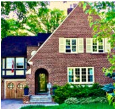
69 Middle Gate, 1926 - evolving versions of the style use red brick or stone for exterior cladding instead of traditional stucco. An asymmetrical design with an off-centre front entrance and a steeply-pitched roof are more identifiers of Tudor Revival.
