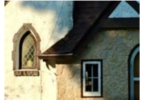
14 East Gate, 1929 - particular windows may be framed by arches; here, it’s a distinctive Tudor pointed arch in diamond-patterned leaded glass.
